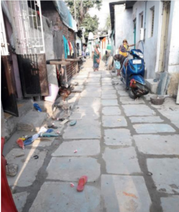
Infrastructure Improvement results in Nagori Vad, Ahmedabad
