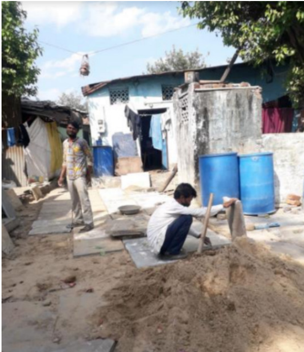
Infrastructure Improvement work in Pirbhai Dhobi ni Chali, Ahmedabad
